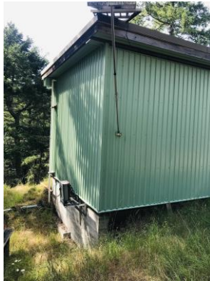
Header Tank Building (side)
