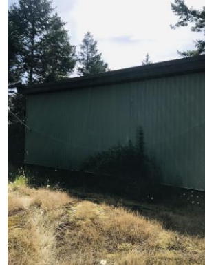
Header Tank Building (front)
